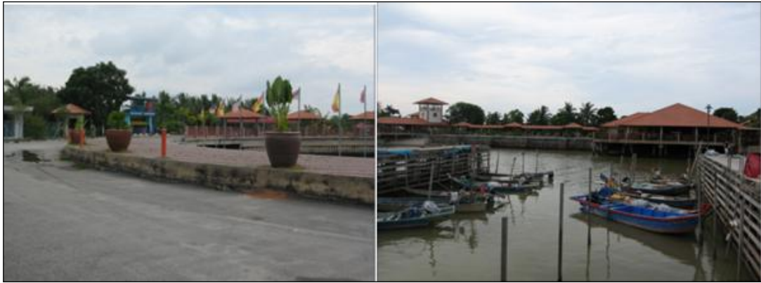
Figure 2.1: Tidal gate and jetty near the Sungai Haji Dorani Rivermouth.
