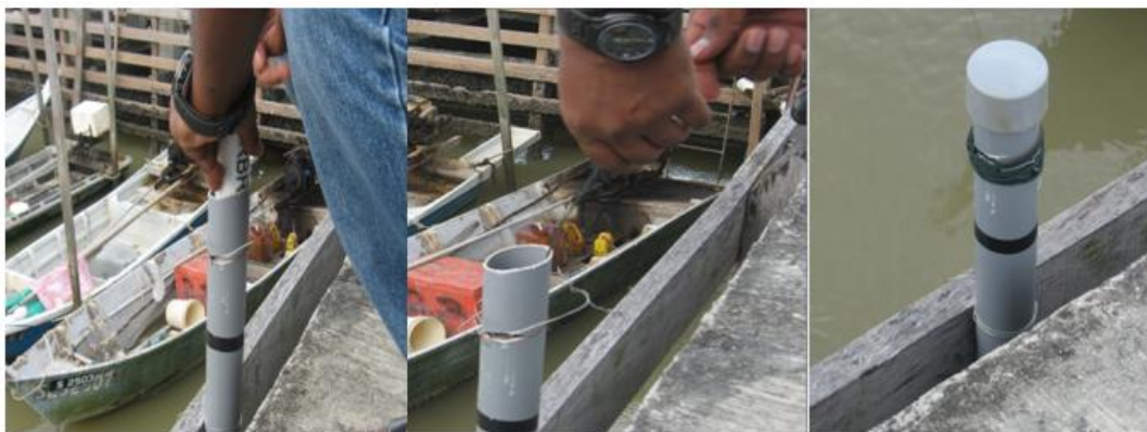
Figure 3.4: The tide gauge TGR-2050 installed at Sungai Haji Dorani Resort. It was secured in the PVC pipe (left) and lowered into the water column (middle). The pipe is then tied to the jetty pillar to secure it (right).
