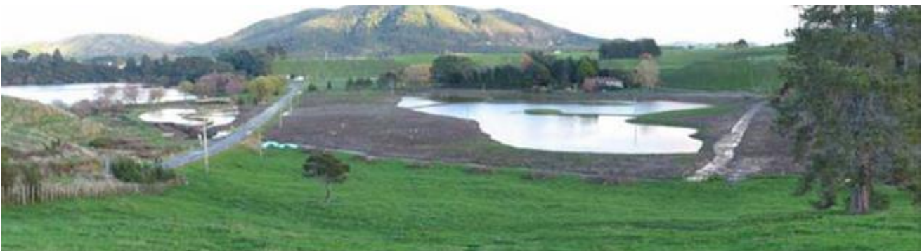
Fig. 34 Wetland soon after completion at Lake Okaro (2005) (LERNZ website)
