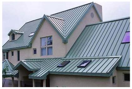
Fig. 1 Long Run Metal Roof
