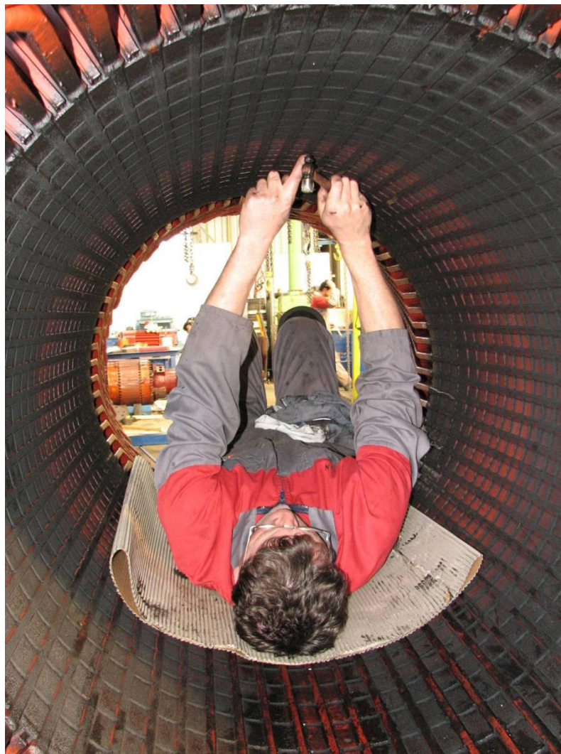
Figure 26: An engineer conducts a Tap Test on a generator armature
