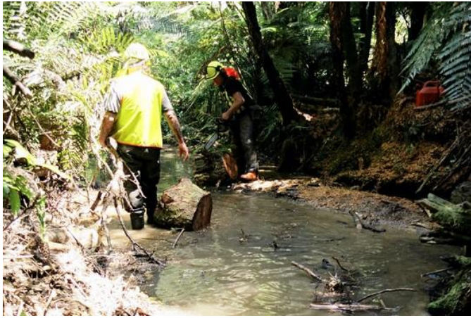
Figure 3.2. a. Wood removal operation in one of the treatment sections.
