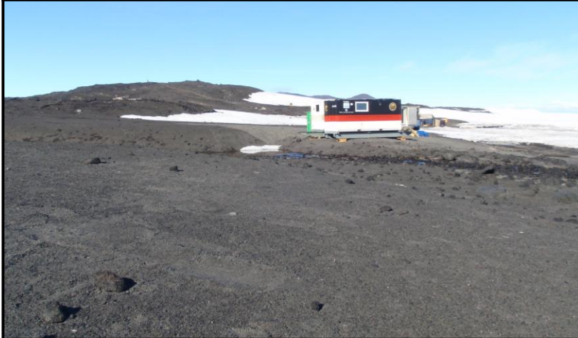
Photo 15: The walk from Home Beach to Terra Nova Hut. Note: AHT workshops and stream.
