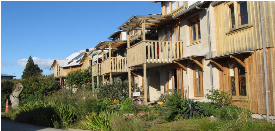
Figure 3: Houses built of rammed earth and natural timber with solar panels visible on the roof
