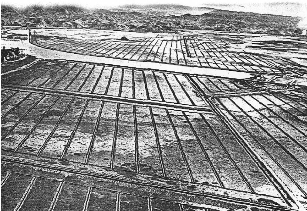
Figure 2.7. Image of the estuary illustrating the construction of the main outfall channel and the extent of the drainage network channels required to make previously inundated land viable for agricultural development. Source: Hawke's Bay Museum.
