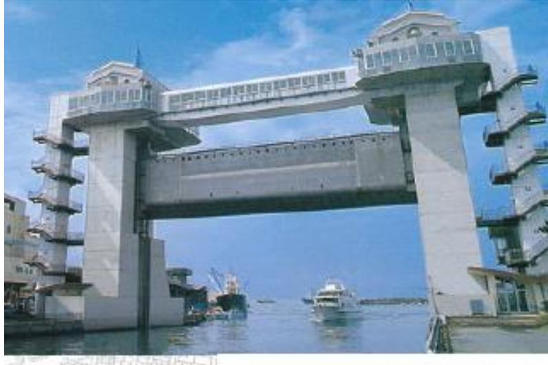
**Figure 63. Tsunami stop gate, Japan.** The gate is constructed at a harbour entrance. The gate height is nearly 10m, the width is 40m, and the gate weighs over 400 tonnes. The gate will automatically close within 5 minutes when triggered by a seismograph signal (Source: Shuto, N., 2007).
