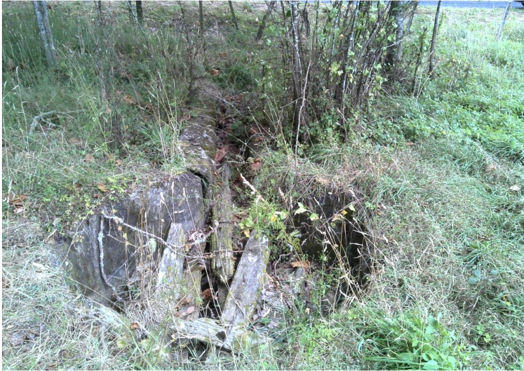
Figure 3-1 Redundant pot bath sheep dip. Last used about 1965. Dip entrance in the foreground and draining pens at the far end of the dip.
