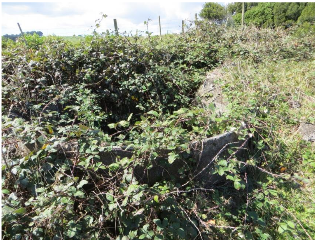
Figure 3-4 Site B, showing the redundant plunge sheep dip with main dip sump in the foreground and draining platform to the left at the far end.
