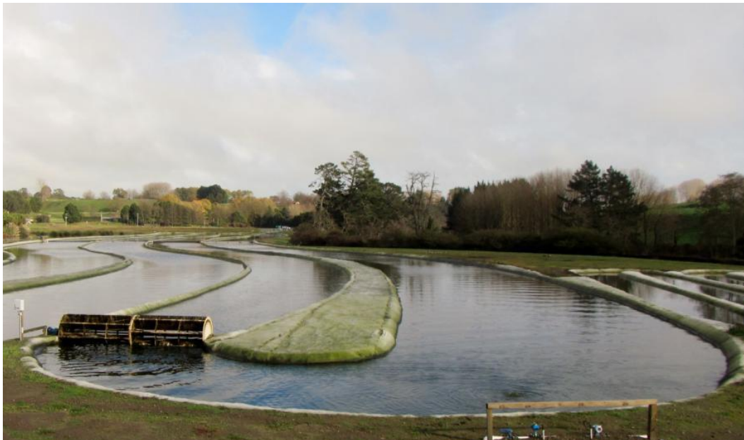
Figure 1 One hectare High Rate Algal Ponds at the Cambridge Enhanced Pond System (EPS). Photo Rupert Craggs (NIWA)
