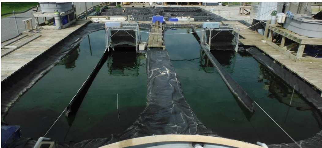
Figure 1 Pilot HRAPs at the Ruakura Research Centre, Hamilton, New Zealand
