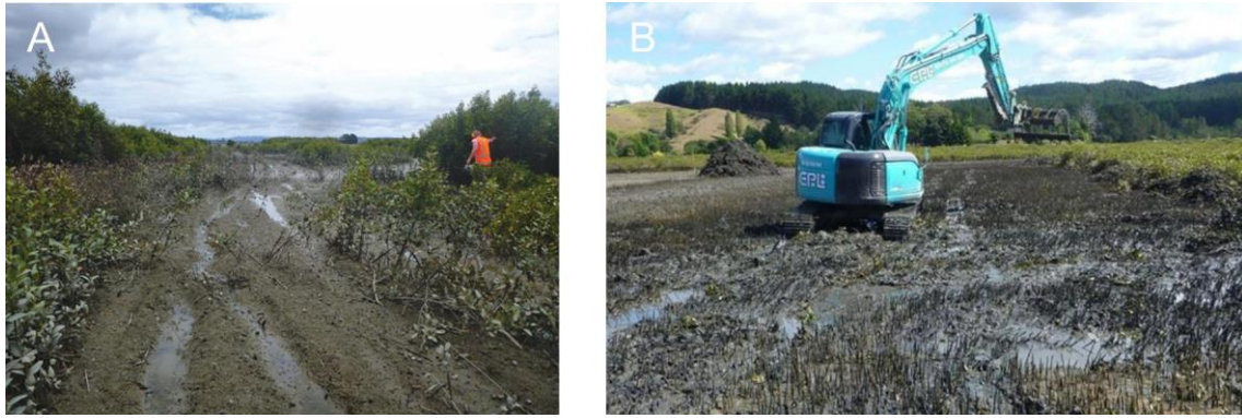
Figure 13. Mangrove clearance in New Zealand: (A) manual mangrove clearance using chainsaws in Mangere Inlet, Manukau Harbour (photo credits: C. Lundquist), and (B) mechanical clearance using digger with rake attachment at Whangamata (photo credits: R. Bulmer).
