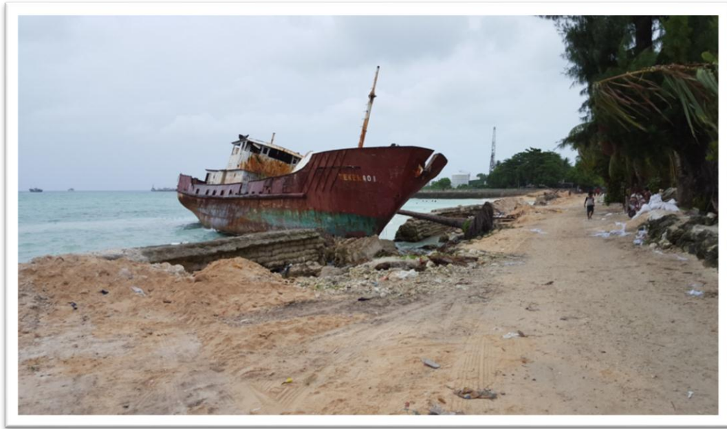
Figure 5.4 Damaged of the sea wall during the 2015 king tides
