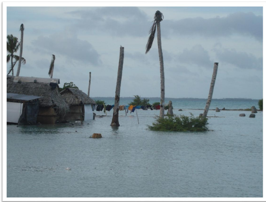
Figure 6.2 Houses flooded by the sea in Eita Village during high tide
