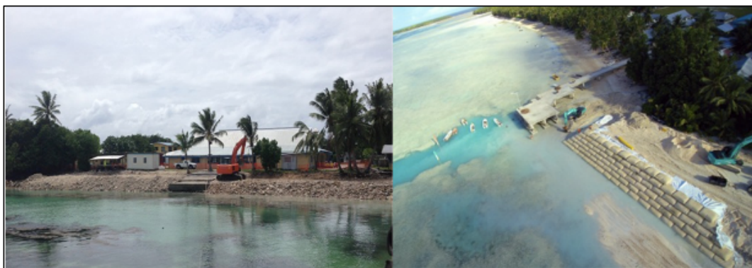
Figure A1.3: Beach nourishment and Geo-synthetic bag seawall in Tuvalu. Source: (Left photo) Courtesy of Apinelu Tili and (Right photo) Used with permission from Newswire website (R) 2 .
