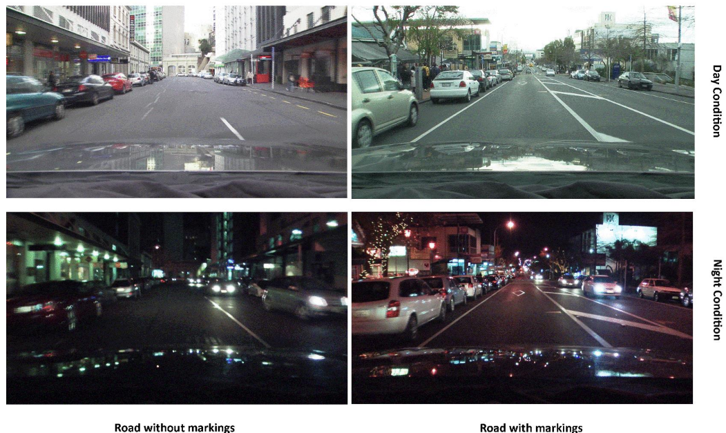
Figure 16: Urban Road Conditions (Day/Night) with Road Markings and Centre and Edge Medians either Absent (Road 1) or Present (Road 2).
