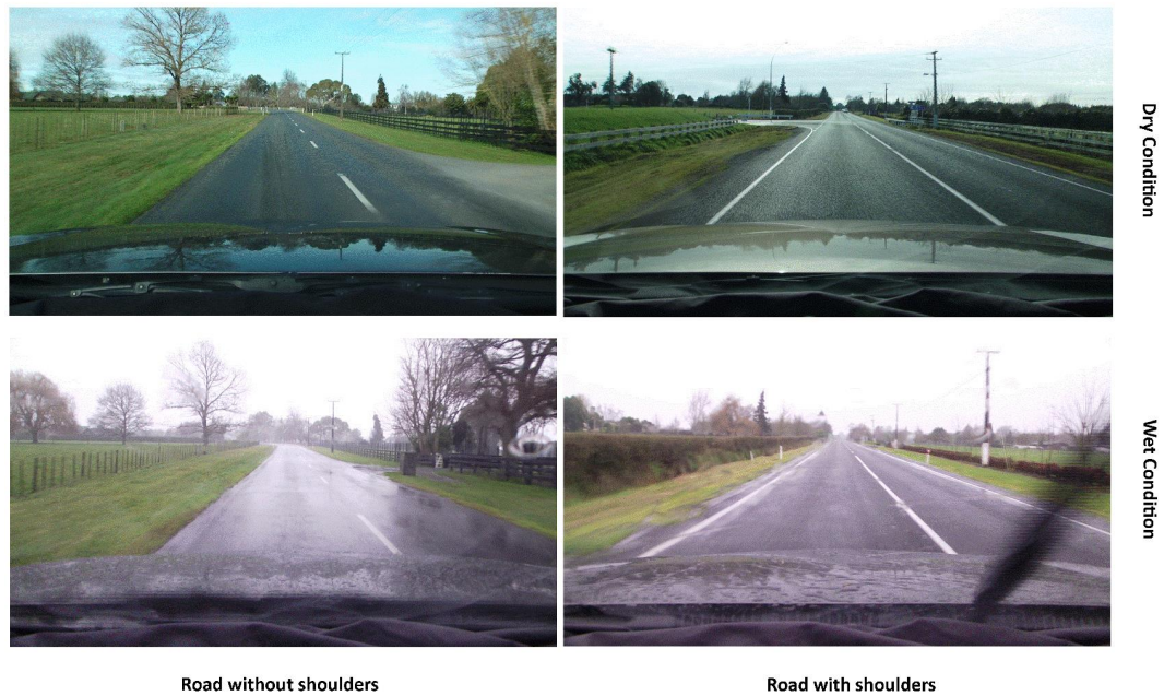
Figure 18: Rural Road Conditions (Wet/Dry) and Types, where lane-markings and shoulder lines are absent (Road 1) or present (Road 2).
