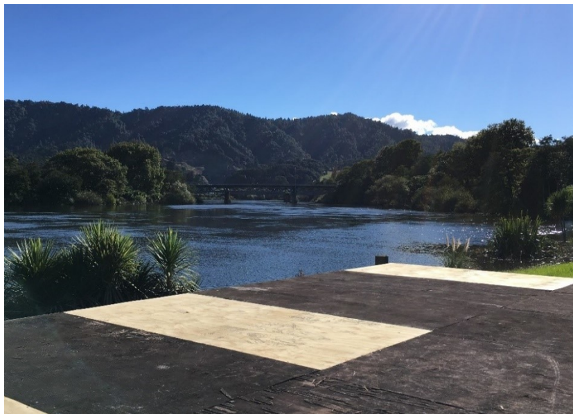
Figure 4. Photograph of the bridge at Ngāruawahia from the barge at Tūrangawaewae marae where an engagement was conducted.
