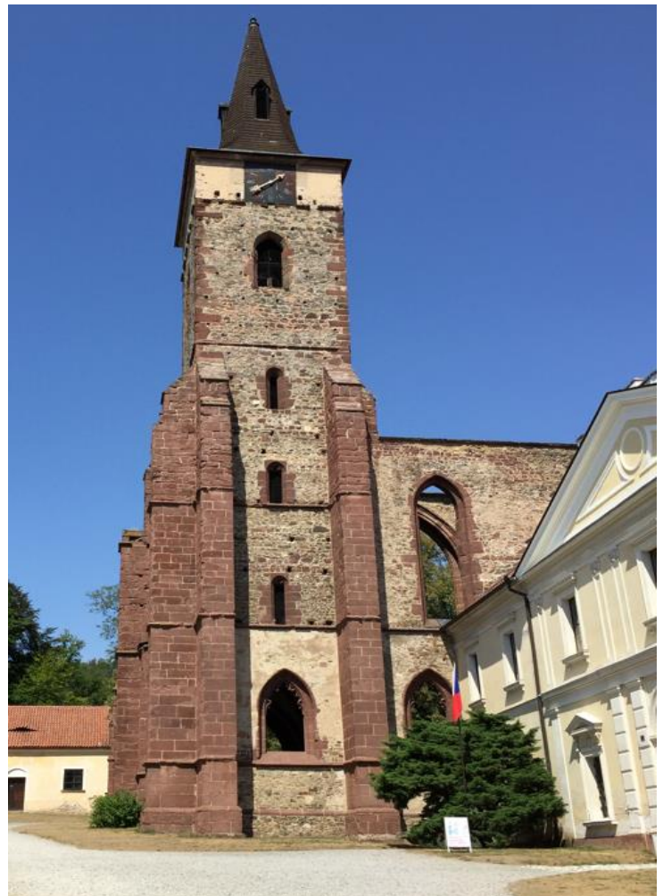
Figure 5.6B – Bell Tower (Present)
