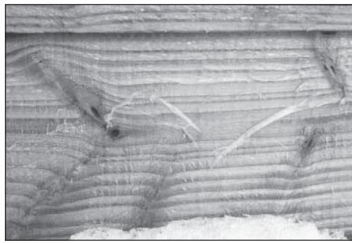
**Non-biological deterioration from Cape Evans hut. Chemical deterioration causing a defibration of wood. As snow melts, large amounts of the wood fibres are removed and the historic wood is gradually destroyed.**
