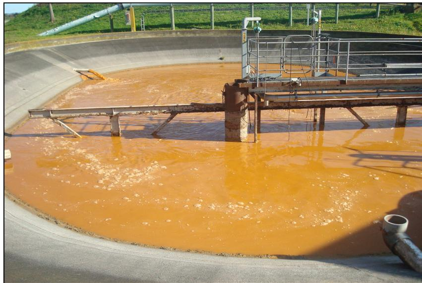
**Figure 4.6** Some of the sludge from the bottom of clarifiers is pumped back to the treatment ponds or disposed off to retain the micro-organisms for the processing at the Waitoa wastewater treatment plant.
