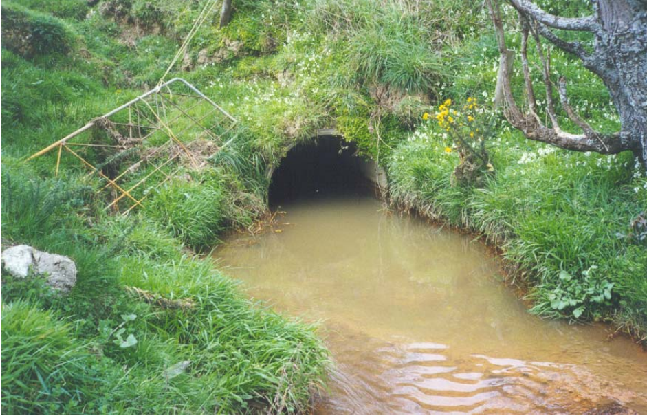
Figure 3. The outlet of the culvert under Sylvester Road on 21 September 2001, showing the drowned invert (photo: Brendan Hicks, 21 September 2001).
