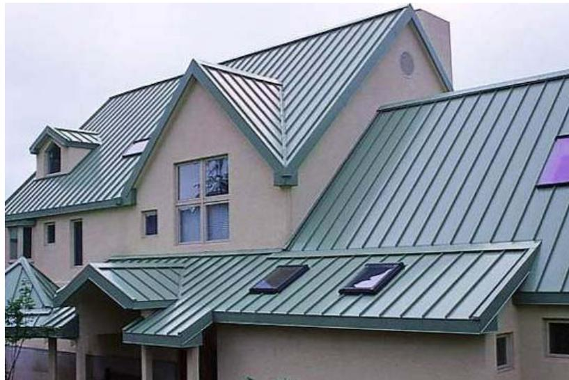
Fig. 1 Long Run Metal Roof
