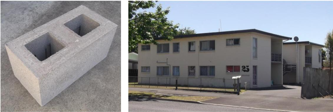
**Figure 5.1: A typical hollow brick used in the construction of apartment blocks in New Zealand, and an example of a ten-unit apartment block<sup>26</sup> (Source: Author)**
