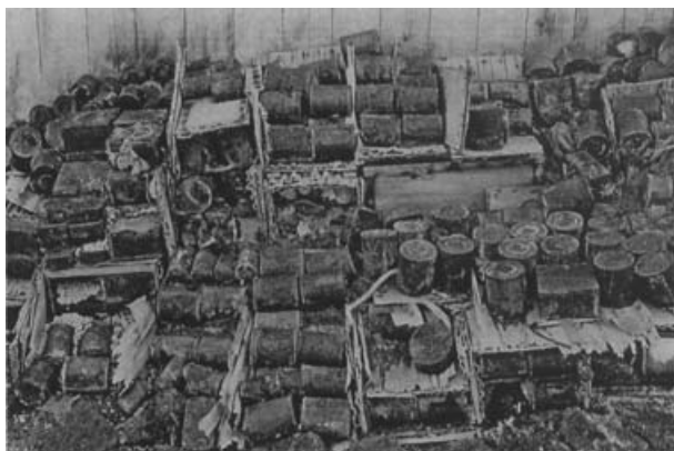
Fig. 6. Deteriorating cans and wooden crates of food stores left at the Cape Royds hut.
