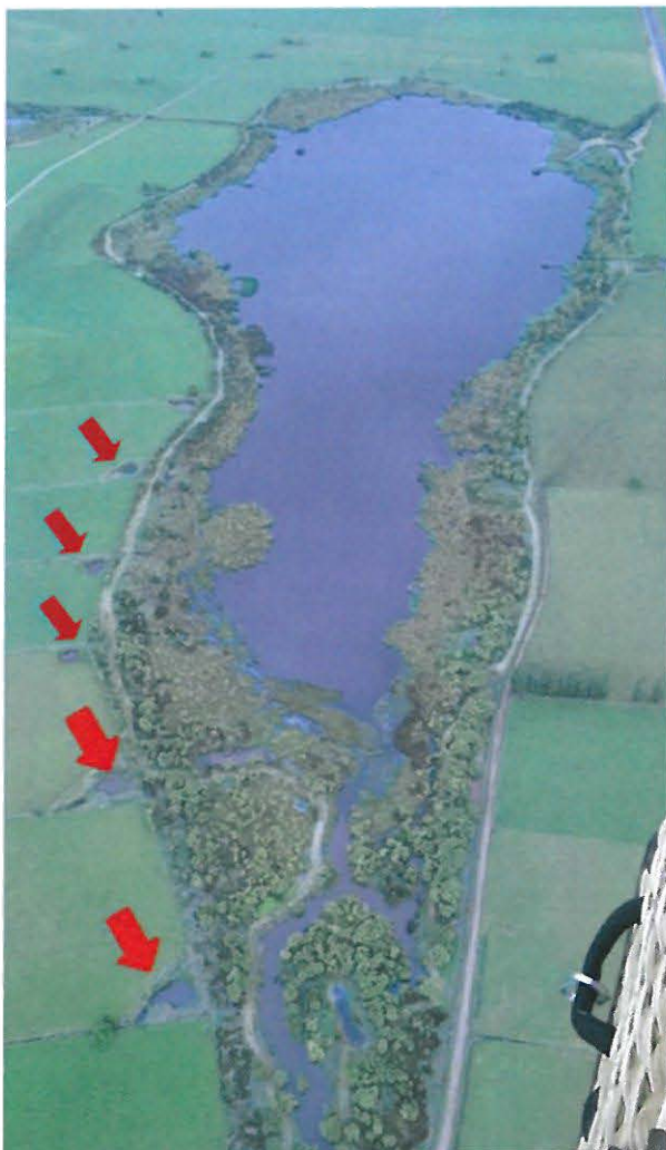
Figure 4. Lake Kaituna. Red arrows indicate sediment detention structures at the end of farm drains.
