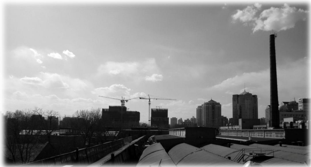
Facing West: Overlooking the factory roofs at 798 Art District with Beijing's skyline in the Background (Author's Research: Allott, 2011)
