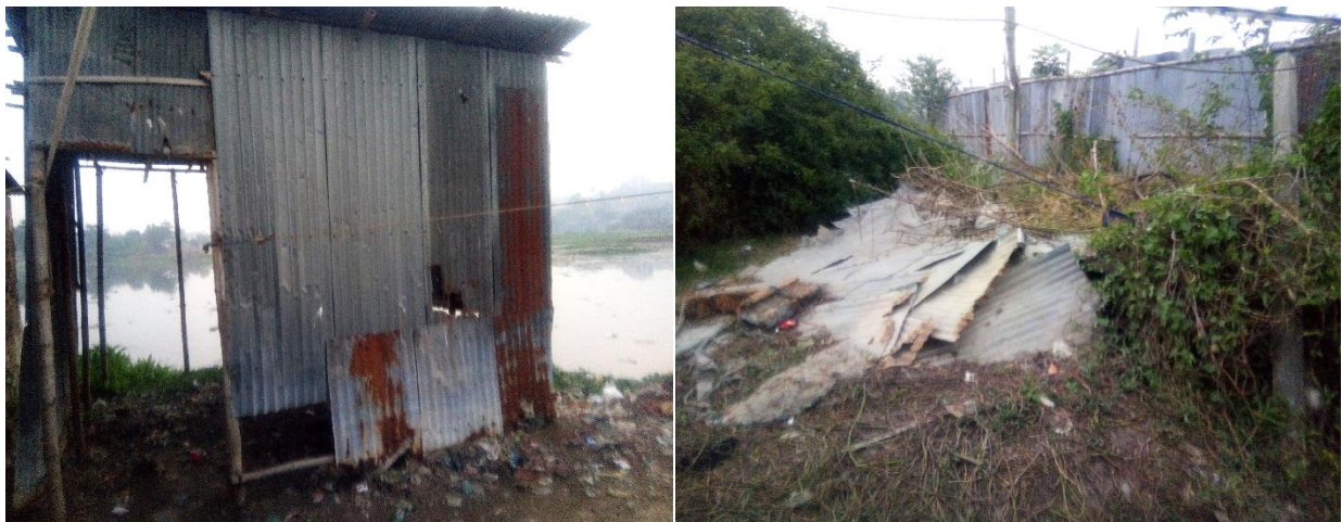
Figure 5.15 and Figure 5.16: Tin-shed houses were blown away by storm near the Lake. Source: Field survey (2018)
