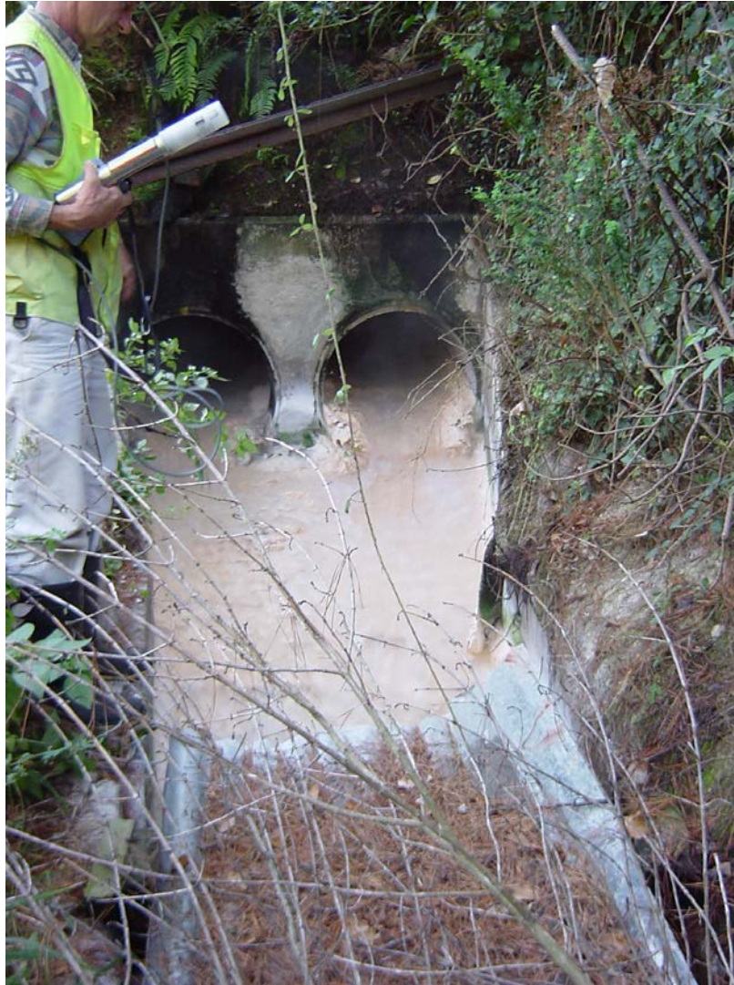
Figure 144. Water for this stream (Site 1) probably sourced from Kiriohineki Stream for the power station (see also Fig. 141). Unnatural silica deposits (well head condensates-no surface waters) are present throughout the stream.
