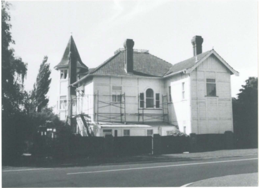
Plate 15 The rear view of Greenslade house, Wellington Street built 1911-1912, undergoing renovation 1988
