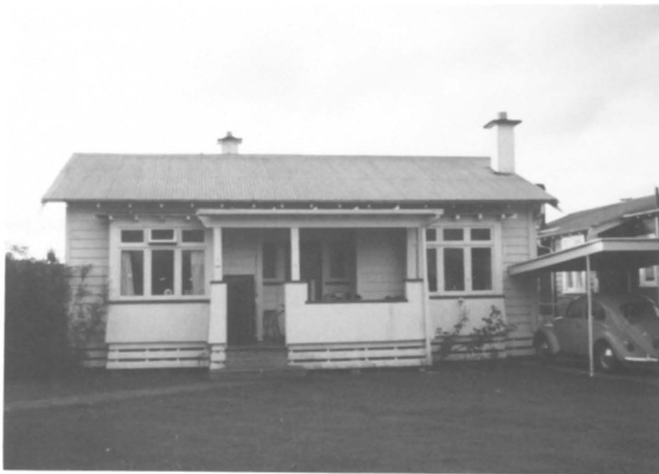
Plate 21 Bungalow cottage in Albert Street
