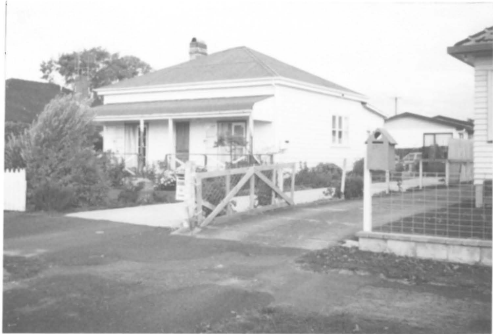
Plate 13 Renovated 1916? square villa, Albert Street
