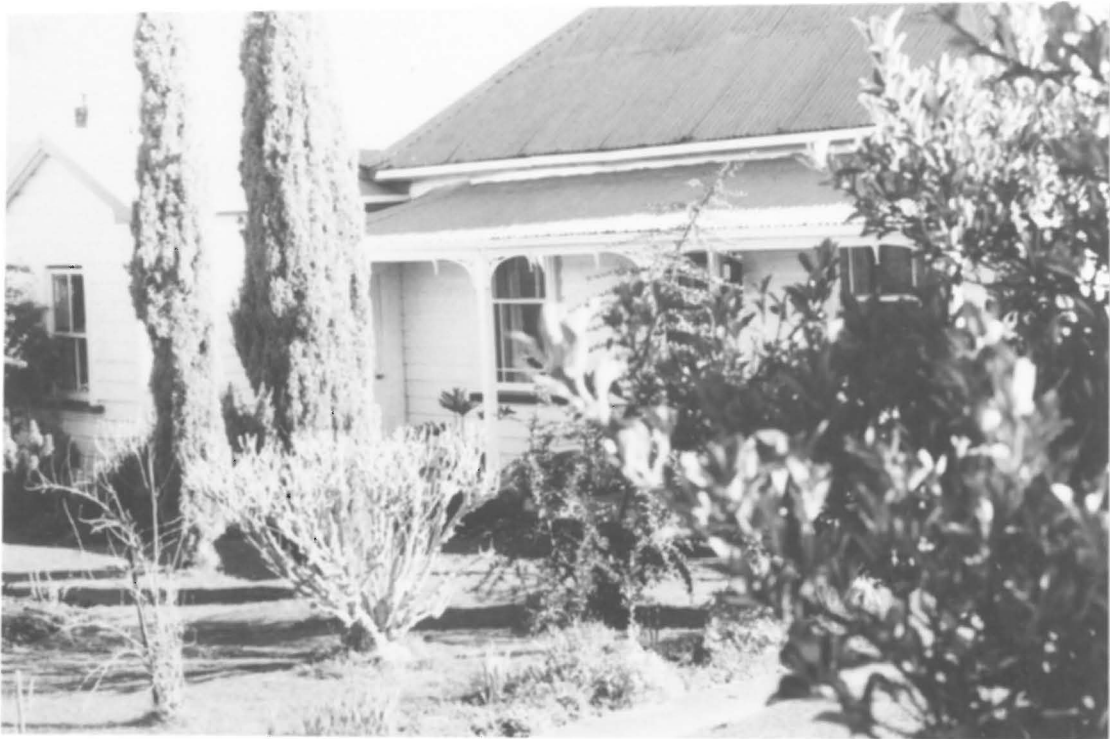
Plate 7 Pre-villa cottage, Galloway Street built c. 1886
