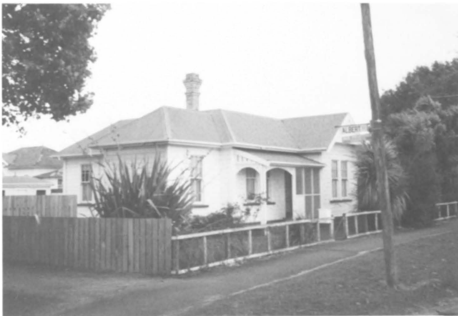
Plate 6 Police station house, Grey Street built 1880
