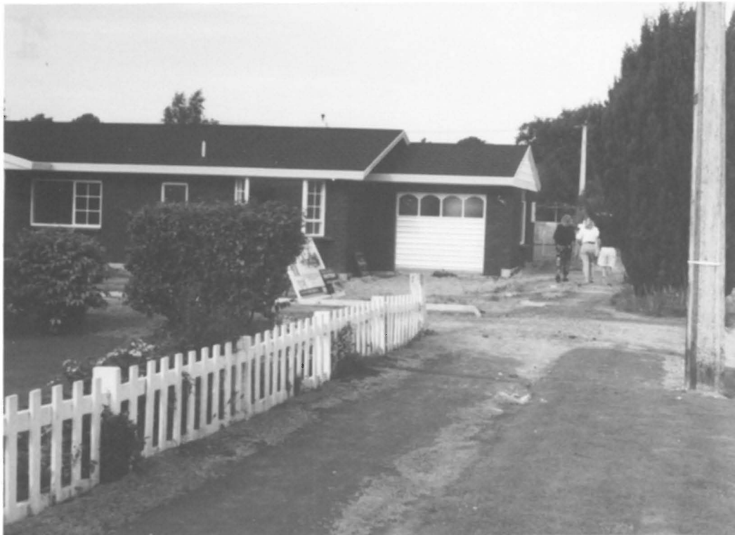
Plate 36 Townhouses under construction in Naylor Street 1990
