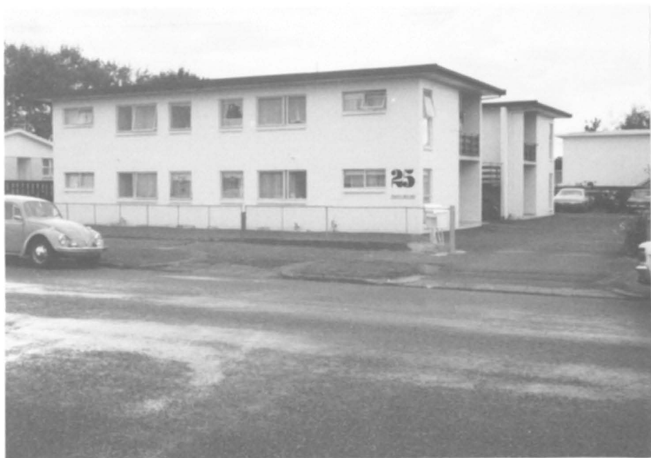
Plate 31 Two storey blocks of flats, Wellington Street
