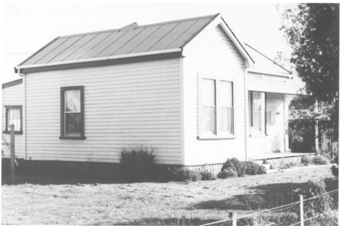
Plate 8 Pre-villa cottages, Wellington and Clyde Streets built c. 1900
