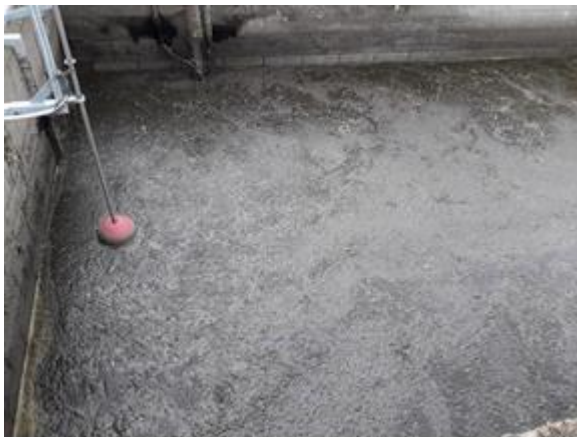
(c) Sump – collection point of Influent sample to the CAP
