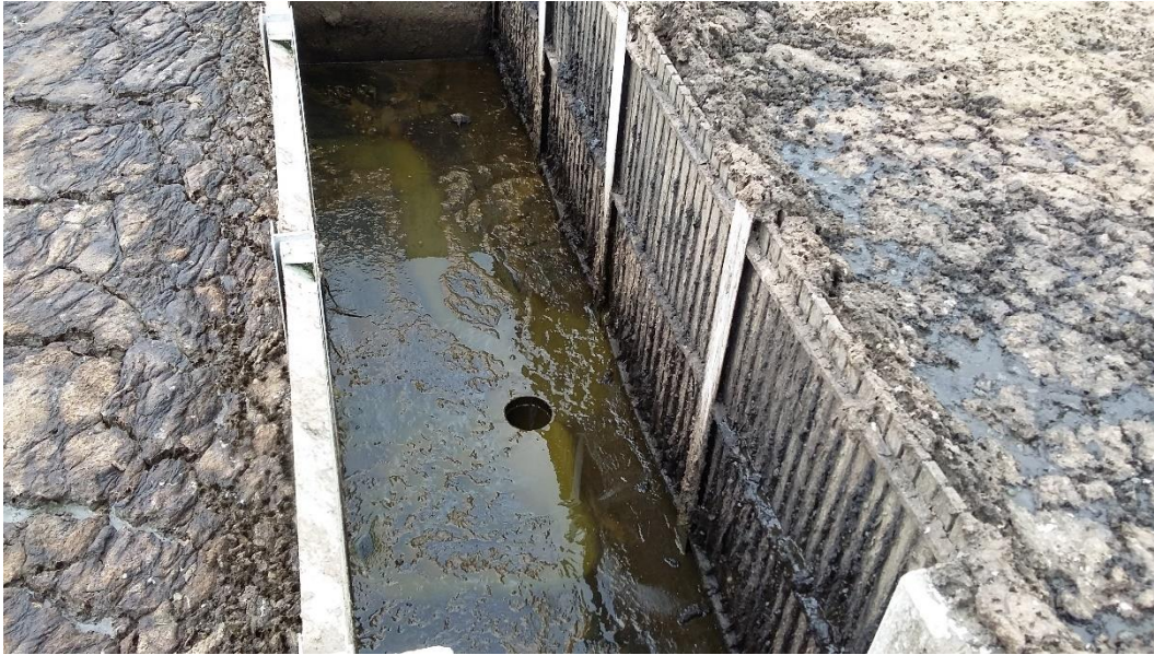
Figure A-4: Passive separator – weeping wall system
