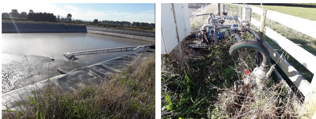
Figure 6-1: Photographs of the storage pond (at approximately 30% full) and discharge pipe.
