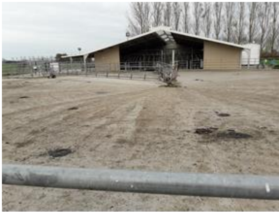
(a) Dairy Shed with milking yard in the foreground
