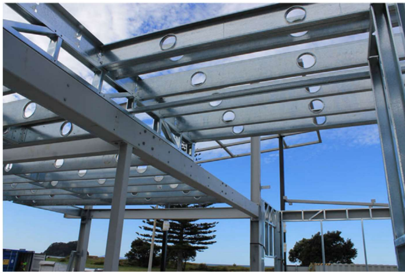
Figure 1.2: CFS channels with edge-stiffened web holes used in buildings [7]
