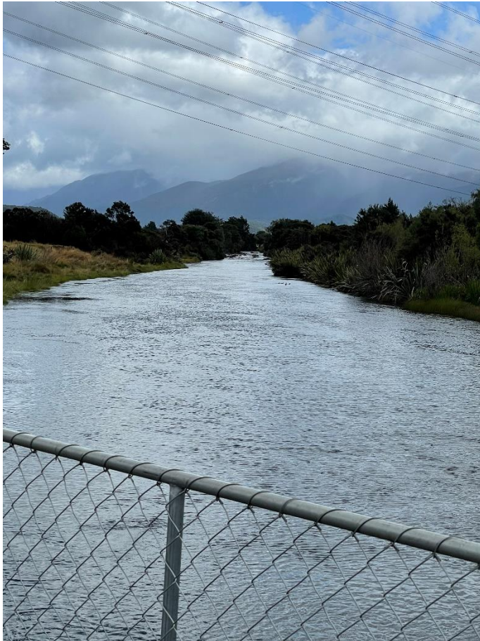
Figure 4.1 Start of Monowai power station headrace (Source: Yasaman Karaminik).
