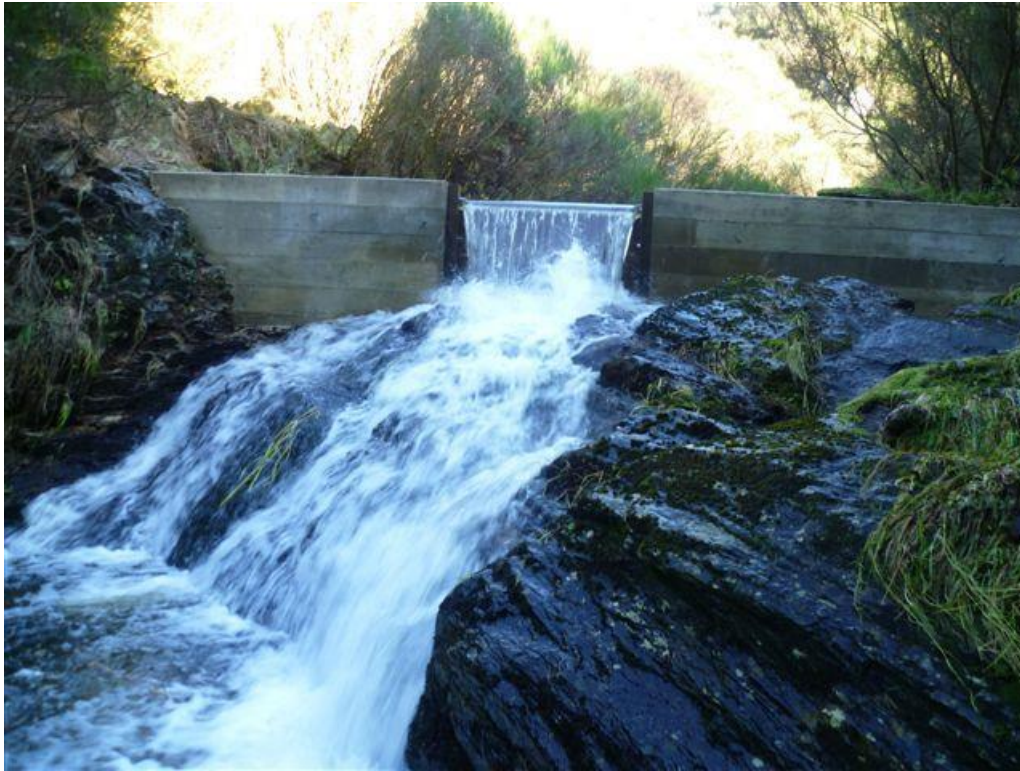
Figure 3.6 Akatore Creek barrier in Otago. A built barrier has been installed onto a natural waterfall to protect Taieri flathead galaxias, after brown trout gained access upstream when conditions changed (Source: Department of Conservation, 2018).
