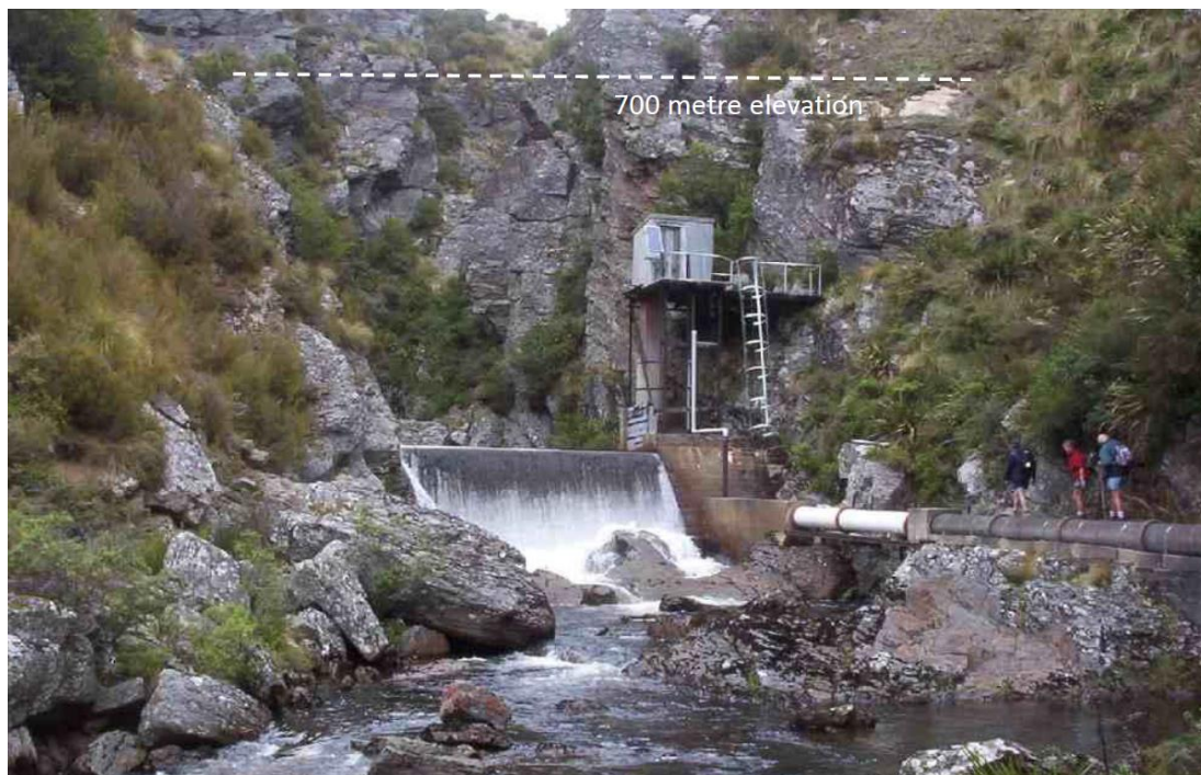
Figure 5.15 Deep Creek Dunedin city water supply intake point. The approximate 700 metre elevation is also indicated. (Source: Taieri Recreational Tramping Club).
