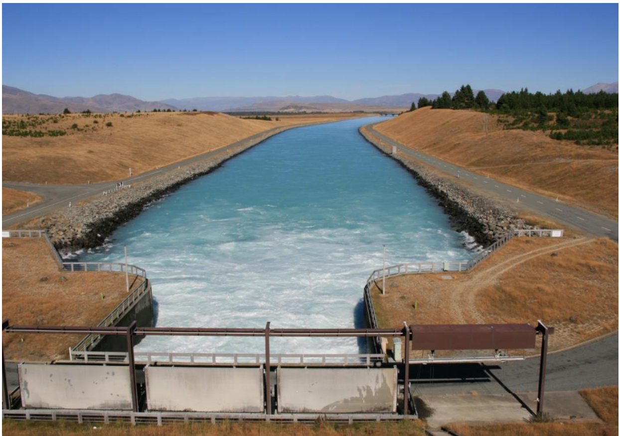
Figure 1.3 Release of water into the Pukaki hydro canal from Lake Pukaki. The canal water previously flowed down the Pukaki River (Source: Mark Oliver Dittrich).
