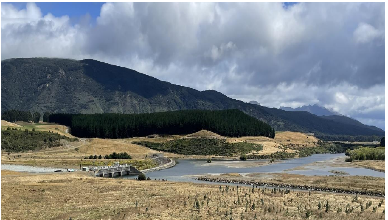
Figure 4.27 Depleted Waiou River (gravel zone on left) visible downstream of the Waiou River control structure at Mararoa. (Source: Yasaman Karaminik).
