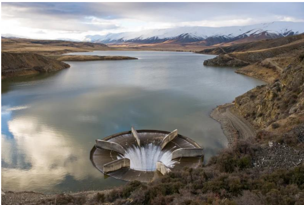
Figure 4.23 Morning glory spillway with water loss from the Falls Dam reservoir (Source: Bill Hatcher/ National Geographic Stock).
