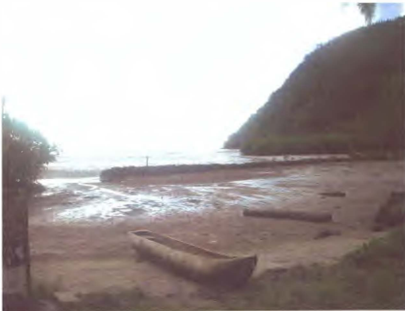
Figure 15 The partly-completed seawall at low tide (Source: Cagilaba 2004)
