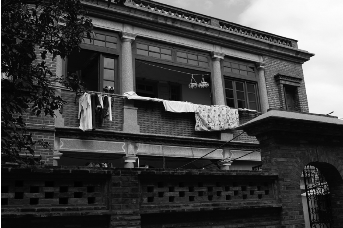
Plate 13: Building with Tuscan columns
