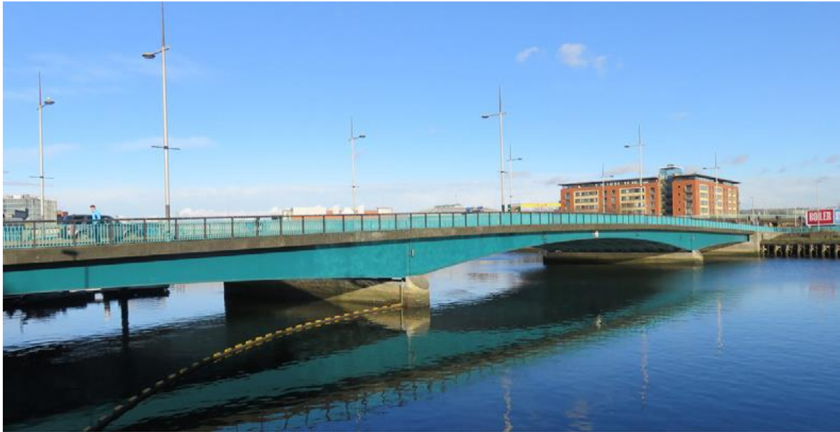
Figure 3 Queen Elizabeth II Bridge (steel continuous girder bridge), Belfast [5].
