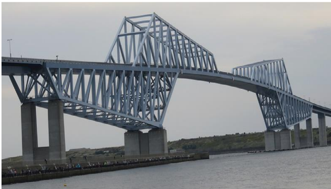
Figure 1 The Tokyo Gate Bridge. (Photo by Lin.) [5].
