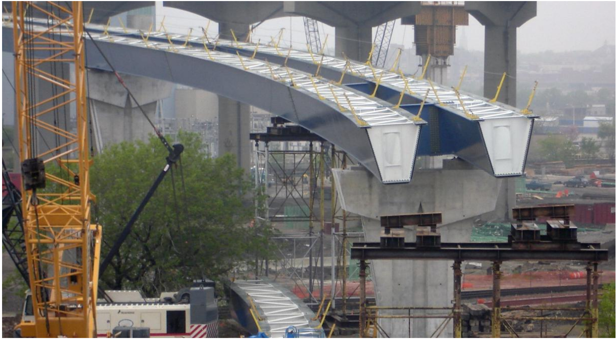
Figure 63 Shows tub girder bridge under construction in Milwaukee, WI, USA [63].
