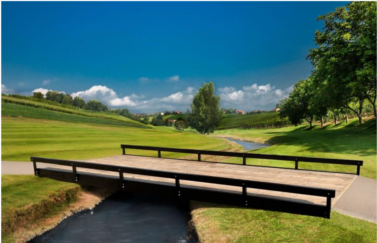
Figure 73 shows steel flat beam bridge [67].
