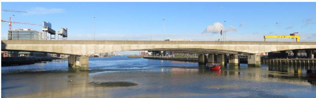
Figure 2 Lagan bridge (concrete continuous girder bridge), Belfast [5].
