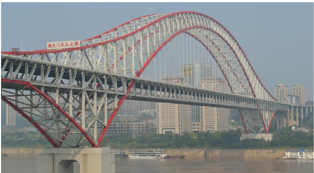
Figure 6 The Chaotianmen Bridge, Chongqing, China [5].
