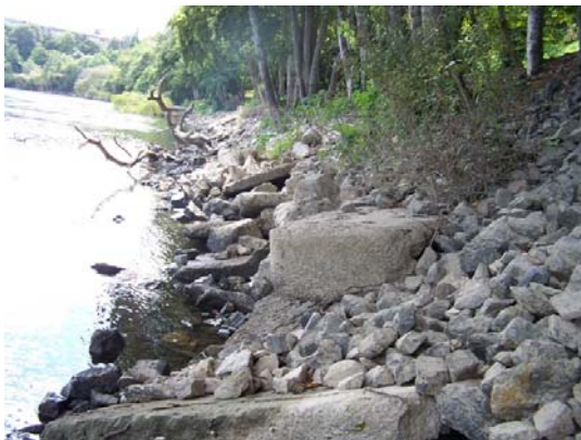
Figure 2.10. Victoria Bridge riprap site showing alder trees spaced along the bank at the top of the picture.
