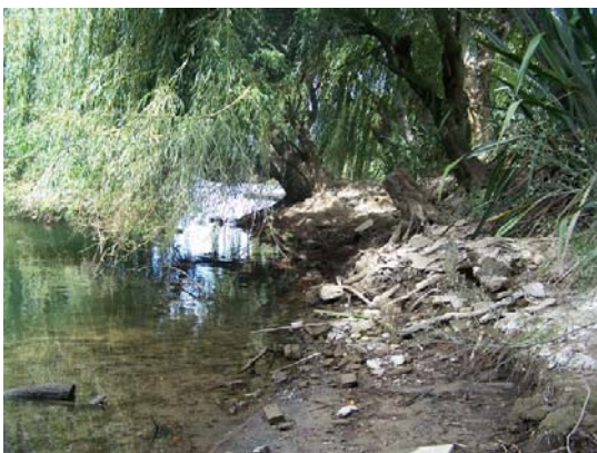
Figure 2.6. Part of Ann Street willow/riprap site showing a weeping willow.
