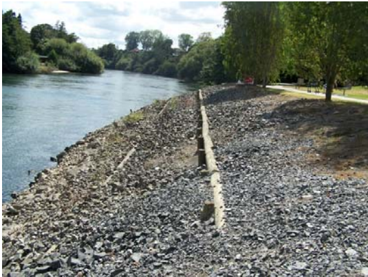
Figure 2.8. Swarbrick Landing riprap site.
