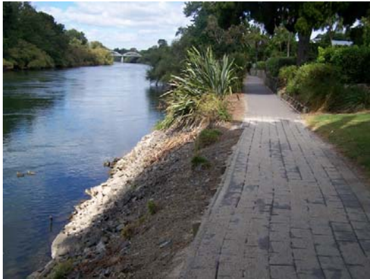
Figure 2.9. Ann Street riprap site looking south.
