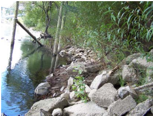
Figure 2.7. Victoria Bridge willow/riprap site.
