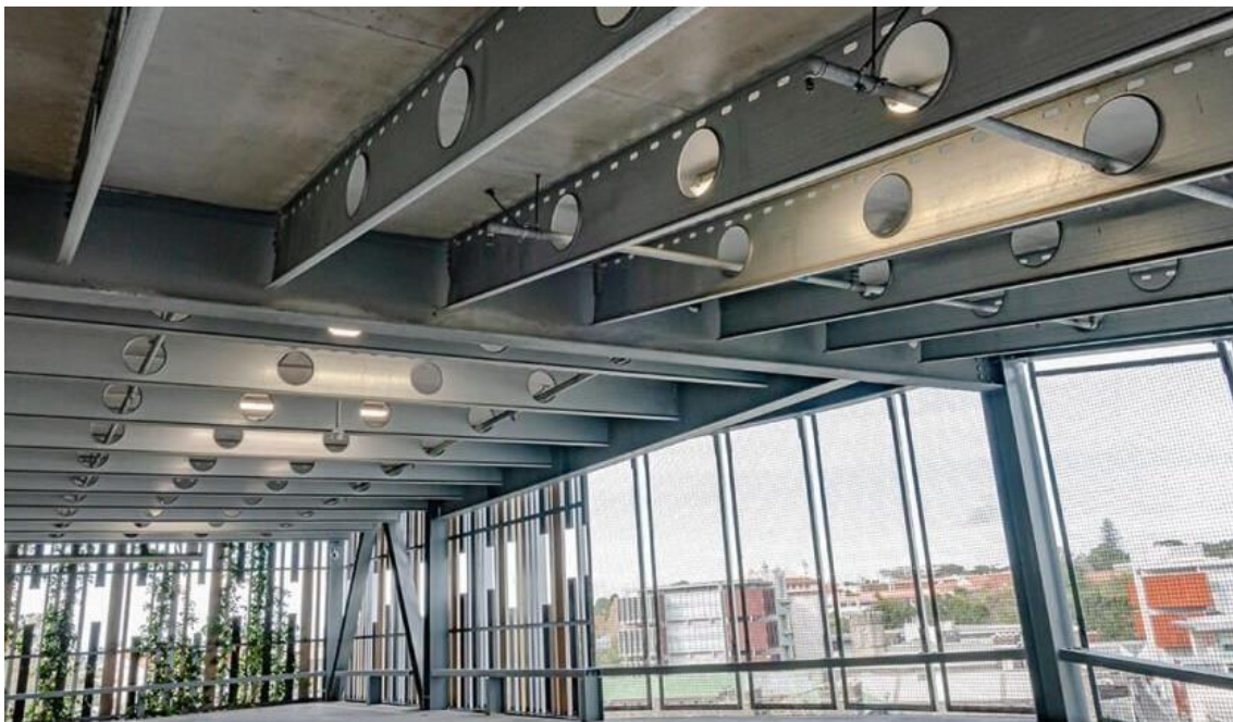
Figure 1-4: Photo of CFS channel beams having edge-stiffened web holes in CFS concrete flooring system [9].
