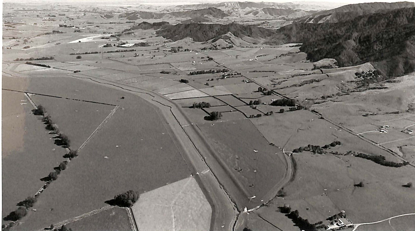
Plate 3.4 : Flood protection works on the Lower Mangawhara River
