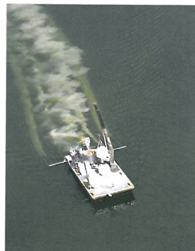
Figure 3. Application of modified zeolite (Aqual-P) to Lake Okaro. Photo: Andy Bruere.
