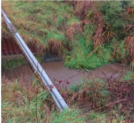
Figure 3.11. OK9 site on bypass channel.
