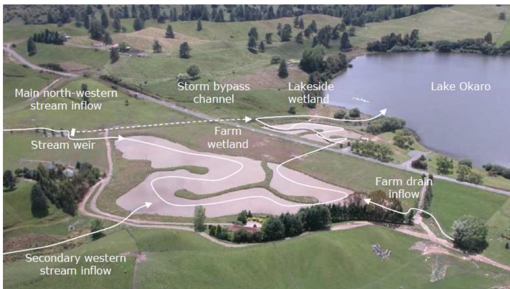
Figure 3.2. Wetland flow path overview, including stream inflows, bypass channel, wetland network, farm drain inflow and outflow. Photo taken after wetland construction, before wetland and riparian planting (Tanner et al., 2007).
