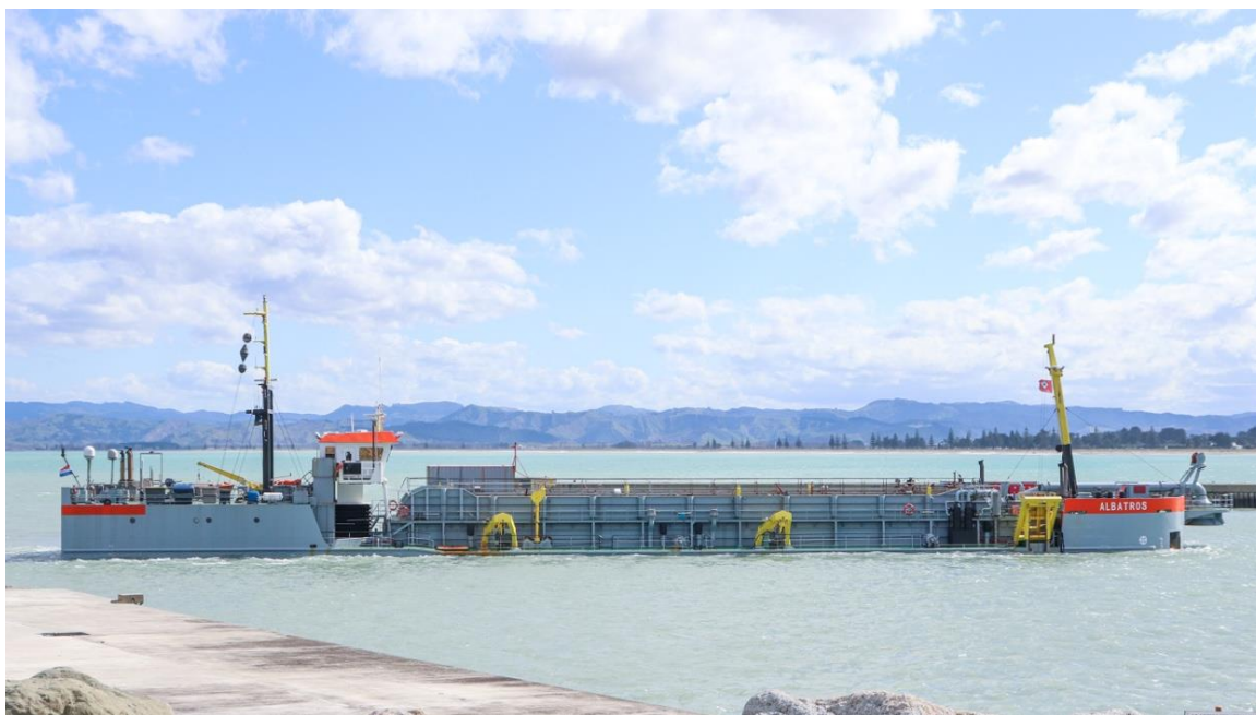
Figure 5-5 Specialist dredging vessel Albatros working in Port Gisborne to deepen the channel.
