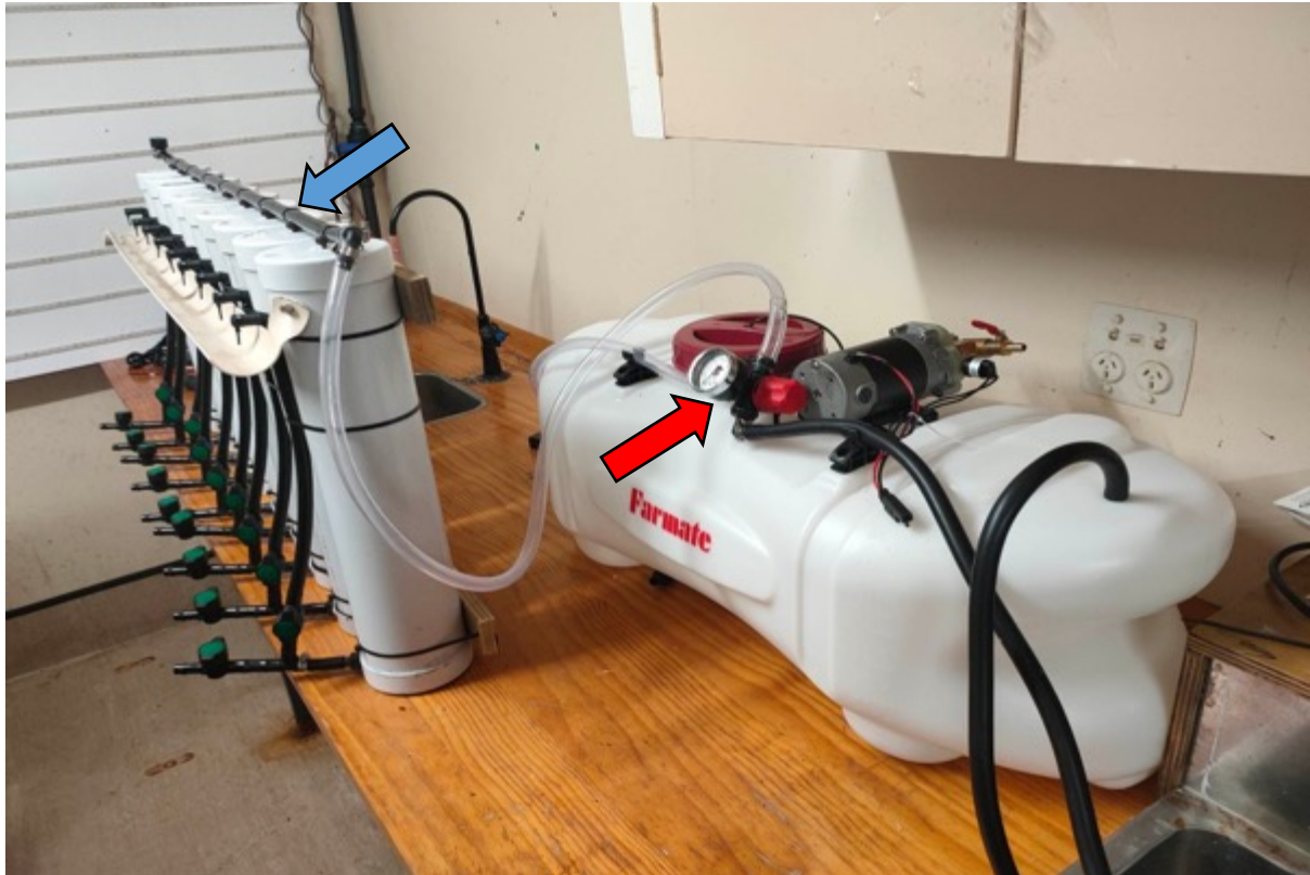
Figure 3. TOPMAQ ATV 12V pump motor and 60-litre Farmate polythene container. Figure 3 Red. Solo 150 psi pressure regulator (red arrow). Figure 3 Blue. Netafim PCJ pressure compensating non-leak irrigation drippers on top of columns (blue arrow).
