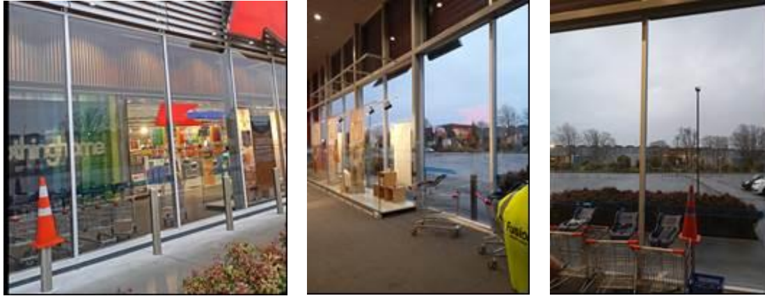
Figure 2-1: The application of aluminium alloy face to face columns used to build glass wall frame for commercial building
