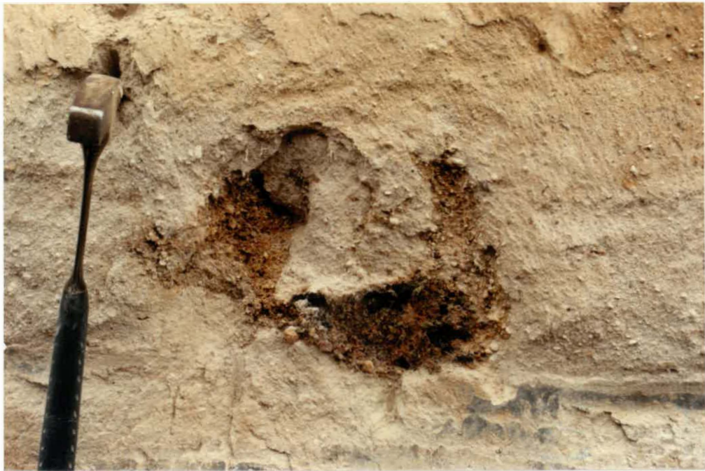
Fig. 3.27 Elutriation of fines by gas given off from the charcoal fragments. Ruahihi Canal (U14/7837270).
