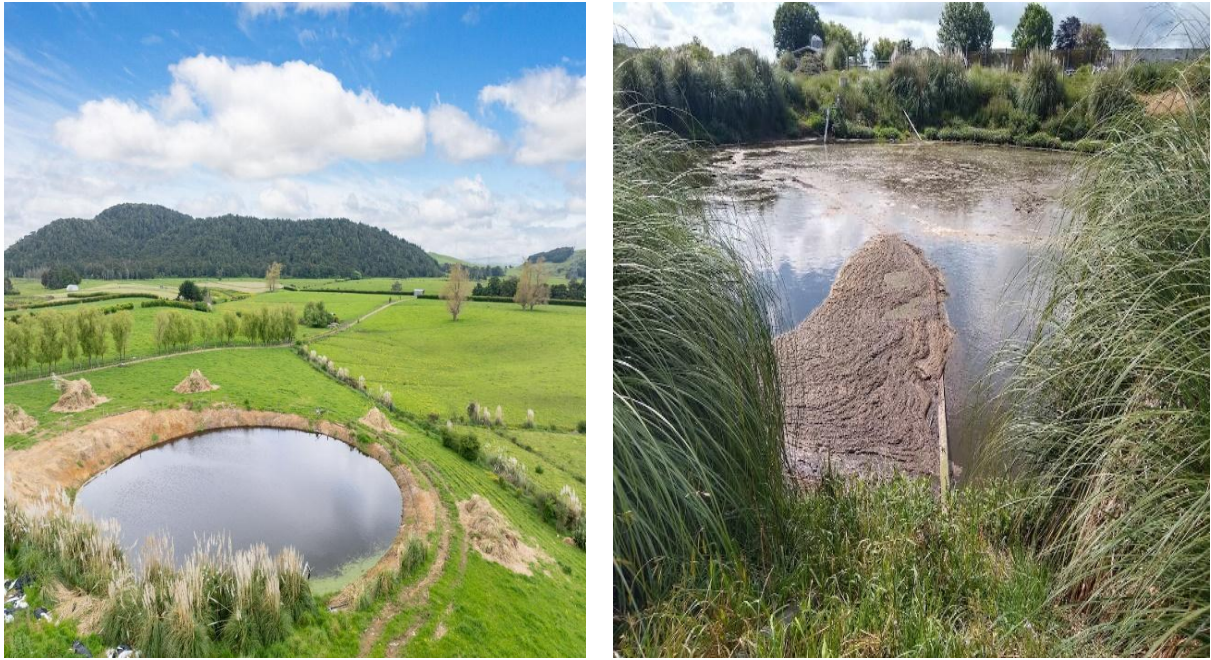
Figure 3-6: The effluent storage pond (images at different angles), where dairy effluent is collected before being applied to pasture as fertilizer.
