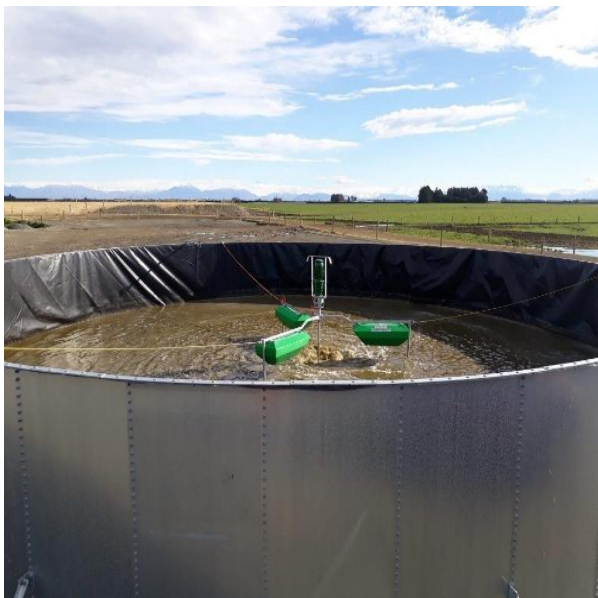
Figure 3-9: Various dairy effluent treatment systems in New Zealand. (Top-left) traditional two-pond system with anaerobic and aerobic ponds; (Top-right) effluent pond at the study site; (Bottom-left) mechanically aerated pond; (Bottom-right) schematic representation of an advanced pond system from (Craggs et al., 2004), including fermentation, high-rate, algal settling, and maturation ponds.
