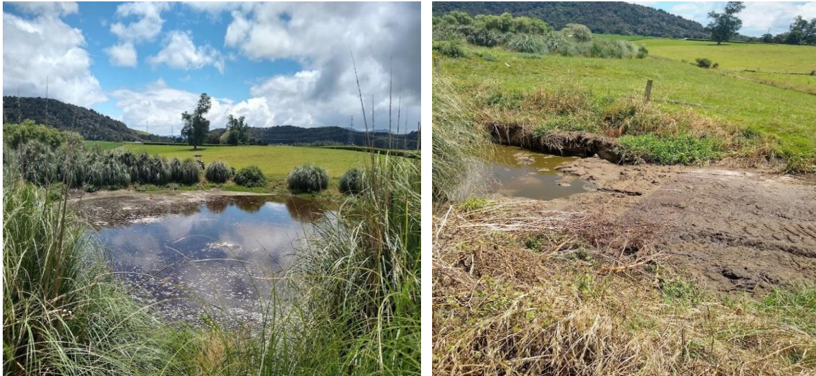
Figure 3-10: Effluent management at the study site. (Left) Effluent pond designed for temporary storage and treatment of dairy farm wastewater; (Right) Stone trapping system at the dairy farm, which helps separate solid materials such as gravel, sand, and organic debris from the effluent before it enters the main storage
