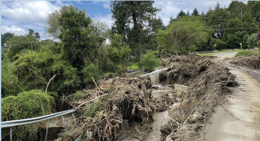
Road damage due to flooding and slip damage near Patoka, Hastings after Cyclone Gabrielle, 17 February 2023, Tania McCauley. Hastings District Libraries 008345. CC BY-NC-ND 4.0
