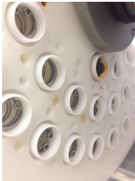
Figure 2.7: Corroded spring on the vial cap.
