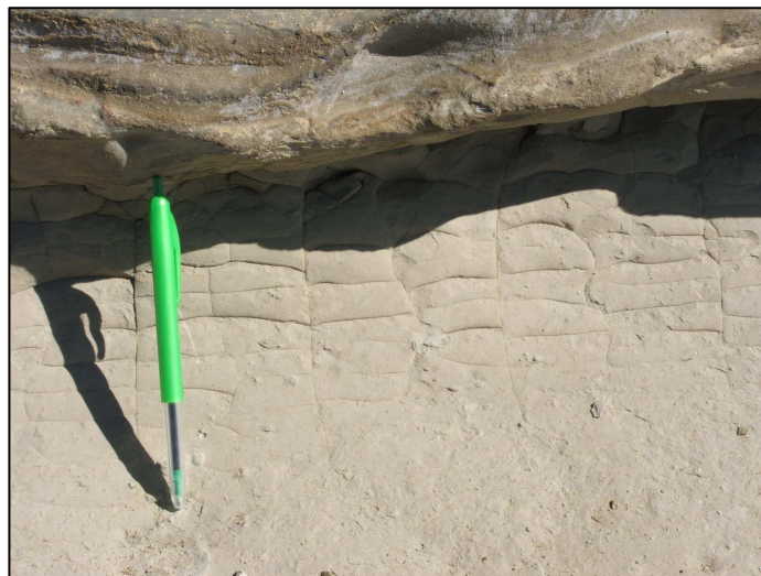
Figure 7.3: Siltstone is more competent at Cockle Bay; the regular closely-spaced joints are still exhibited but loose, curved siltstone fragments that are easily removed from the cliff face are not apparent.
