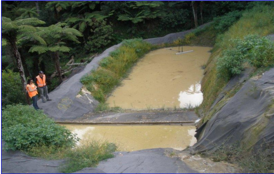
Figure 3.3 Sediment retention pond 8 in April 2009.
