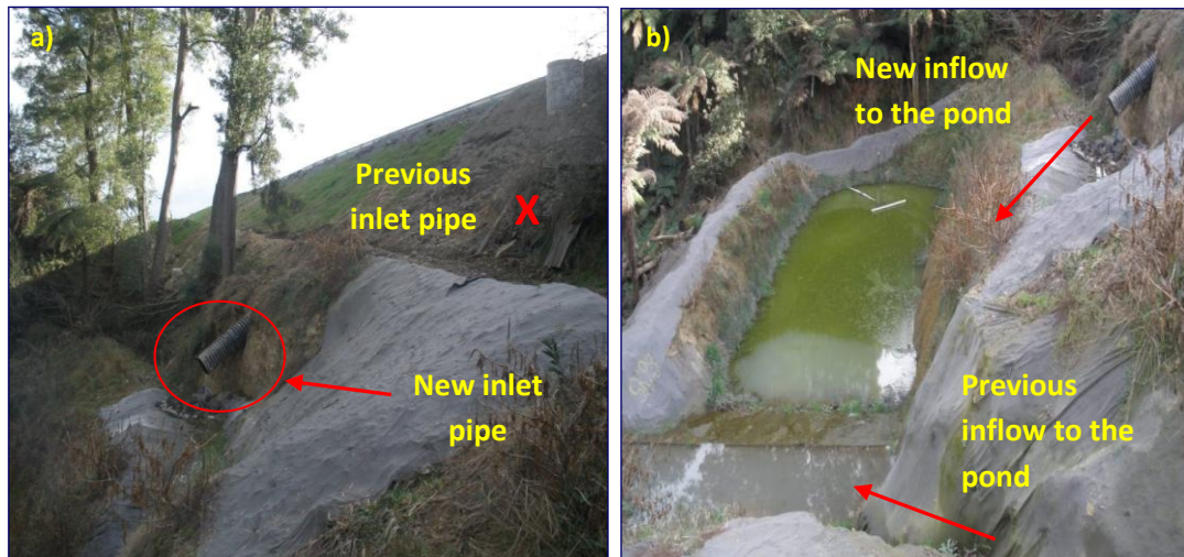
Figure 3.7 a) and b) New inlet installed closer to the pond.
