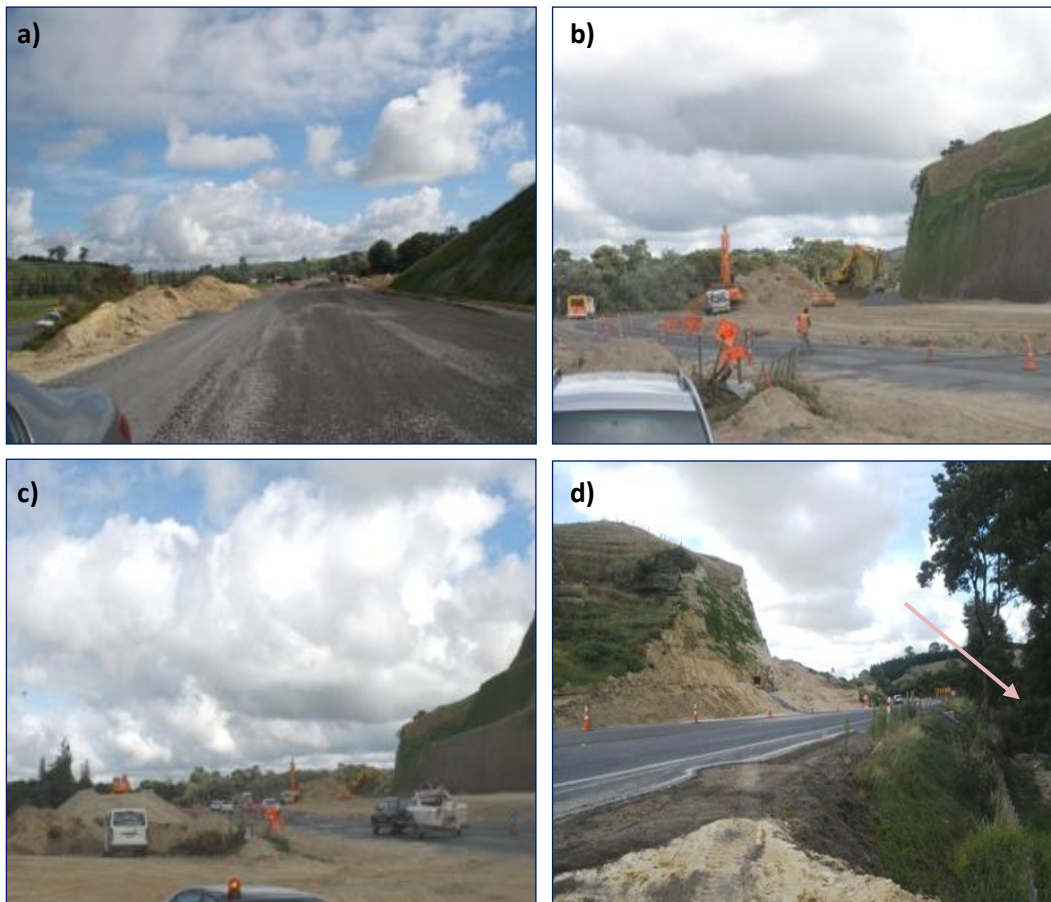
Figure 3.4 Realignment of SH1 to Tirau; (a,b,c) showing the earthwork activities along the 4.5km section of SH1 involved; (d) indicates the catchment of sediment retention pond 8, arrow pointing at the location of sediment retention pond 8.
