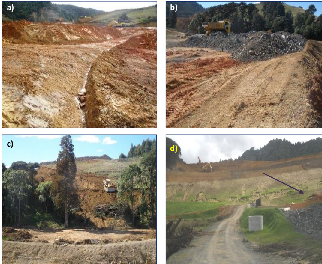
Figure 3.10 Perry's Aggregates quarry Site at Waingaro Road in Ngaruawahia (a,b,c) showing the earthwork activities at quarry site; (d) indicates the catchment area of sediment retention pond 2, arrow pointing at the location of sediment retention pond 2.
