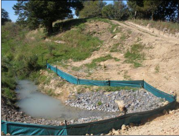
Figure 3.11 Silt fence to prevent overland sheet flow entering stream.
