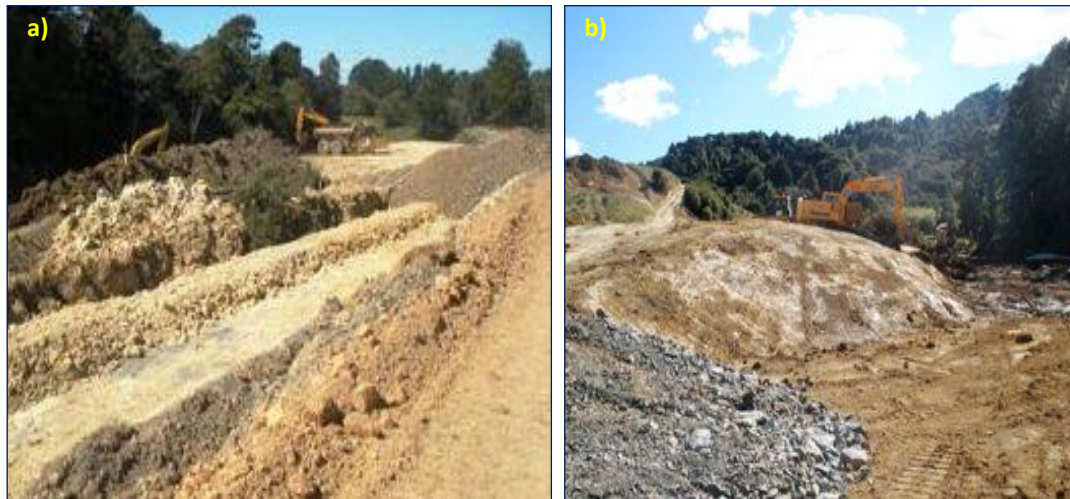
Figure 2.1a and b. Soil disturbing activities on active earthwork sites involved cutting, blading, ripping and compaction of soils.
