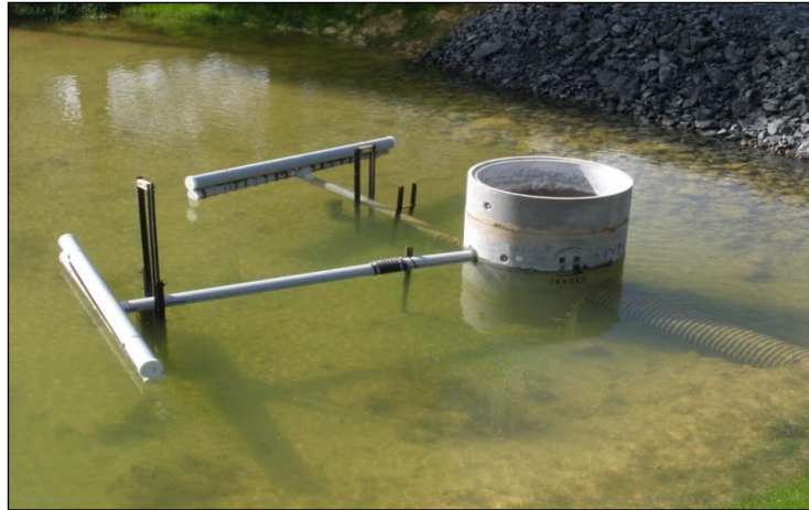
Figure 3.14 Decanting structure of sediment retention pond 2
