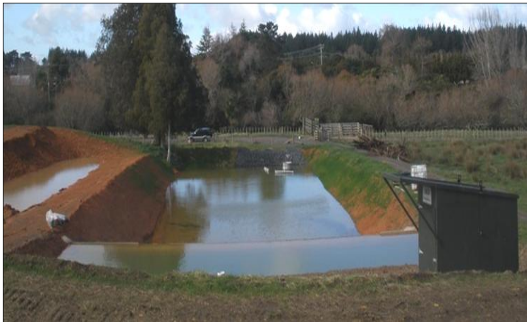
Figure 3.9 Sediment retention pond 2 at Perry Aggregates, Waingaro Road quarry site.
