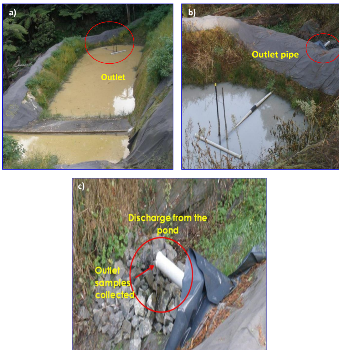
Figure 4.8 a, b and c Discharges from ponds were collected directly from the sediment retention pond's outlet pipe at Piarere.
