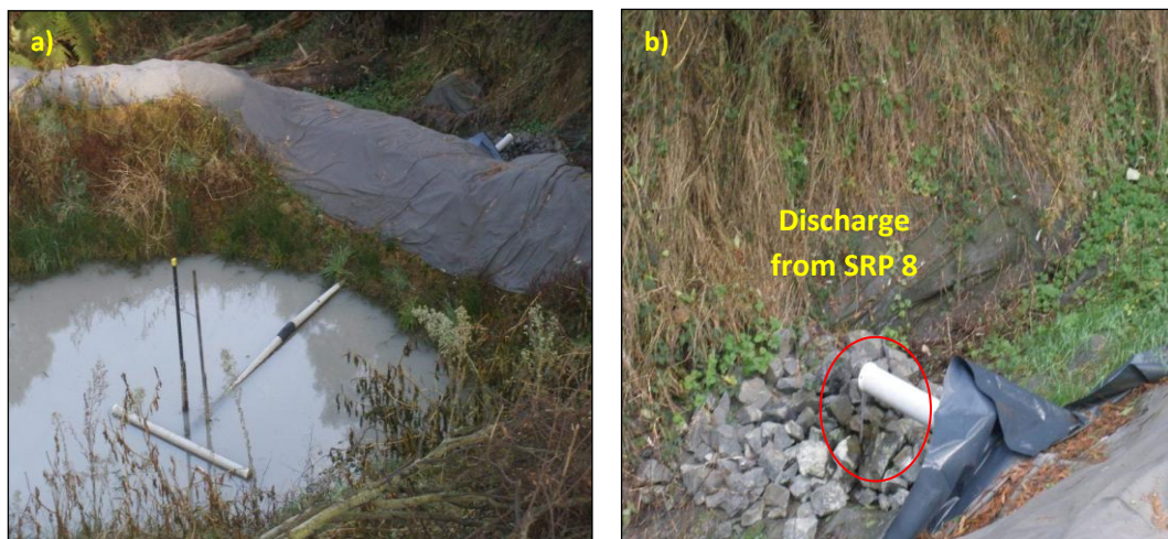
Figure 3.8 a) Decanting structures of sediment retention pond 8; b) Outlet pipe channelling discharge from sediment retention pond 8 to the bush area.
