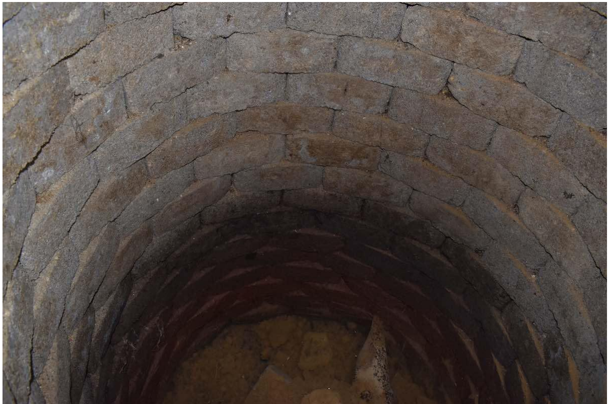
Figure E.9. Photograph showing the inside of the easternmost well.
