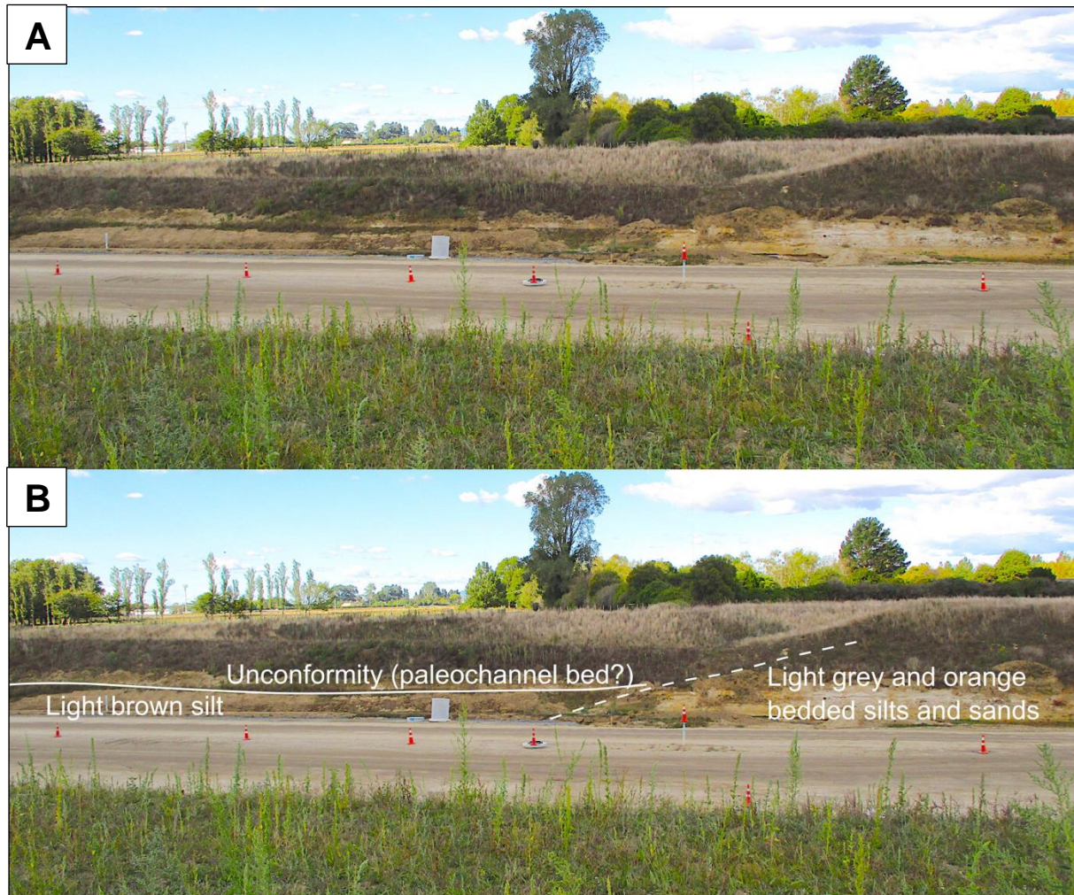
Figure 3.33. Waikato Expressway cutting approximately 500 m south of the Ruakura Interchange. (A) Photograph of the eastern wall; (B) same photograph annotated, showing what appear to be a lateral discontinuity and unconformity – possibly a paleochannel bed – the latter coinciding with perched groundwater given in Beca Ltd (2016).
