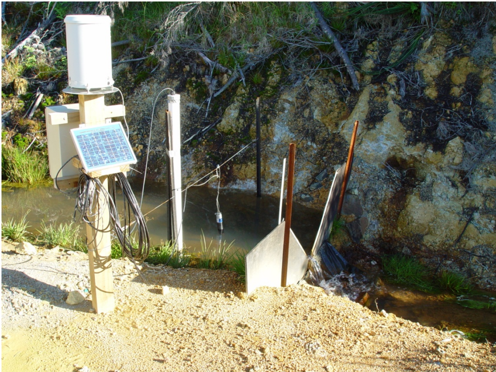
Figure 8.11. EX-H6 site showing the housing for the logger, rain gauge (mounted on top) and the power supply via the solar panel. The OBS turbidity probe was mounted using the suspension method and a low flow condition over the V-notch weir.
