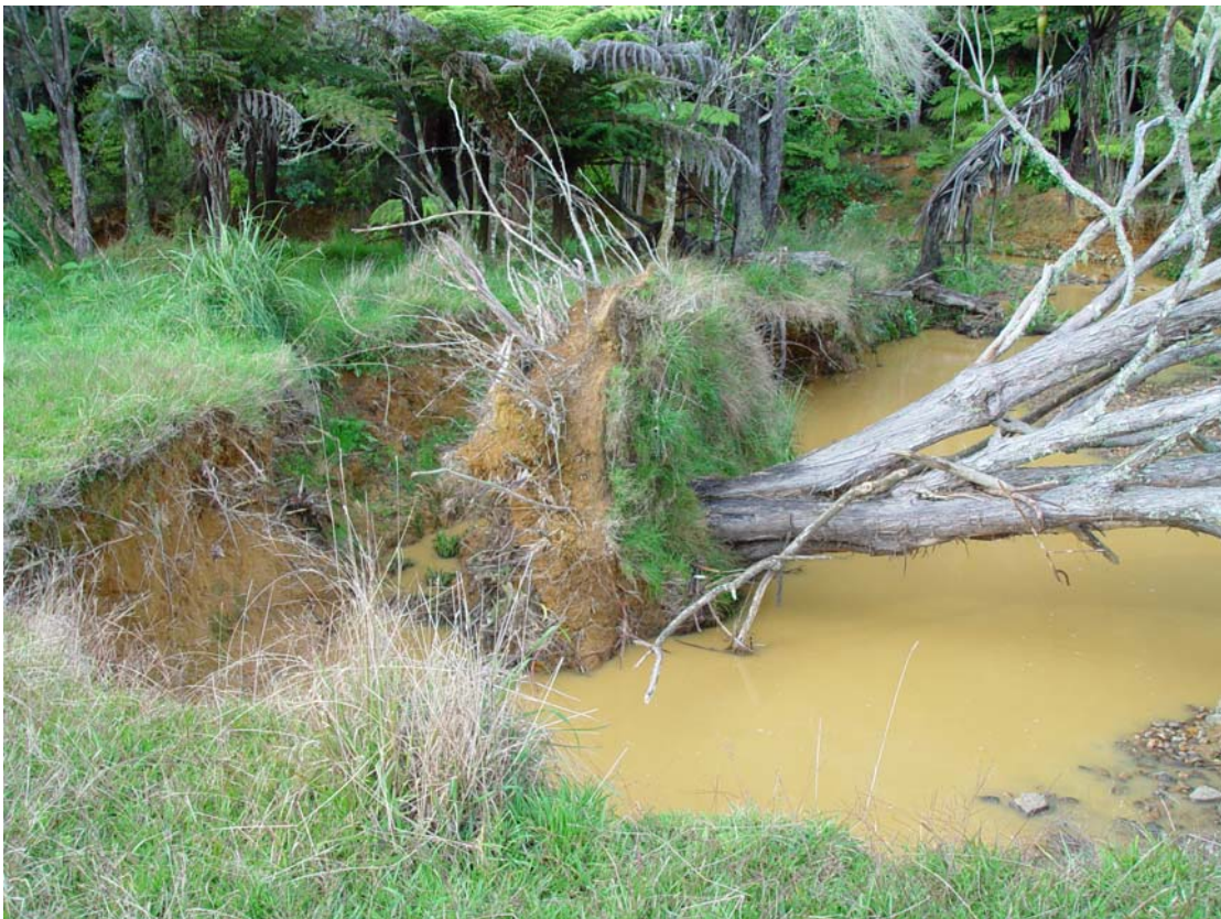
Figure 11.8. Area of streambank erosion in the agricultural landscape unit.
